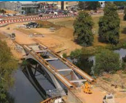
Image: Steel arches erected prior to installation of cross girder and concrete deck slab construction
