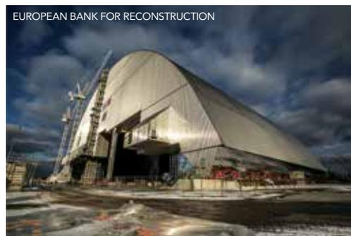
confinement structure has been reached. As seen on national media, an arch shielding the radioactive waste caused by the 1986 accident has started sliding into place.
