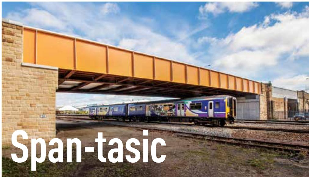
Tony Gee has successfully completed the design of a challenging 11-span overbridge reconstruction at the throat of Bolton railway station.
