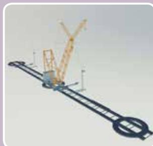
The 500m foundation will support a massive rail-mounted crane specially designed to lift the heaviest elements of the new nuclear power plant. Much of the reinforcement will be prefabricated on-site and lifted into place. Tony Gee has designed the cages to be lifted including reviewing the lifting beams, the reinforcement ties and specifying additional clamps where necessary. Only at more complex intersections is the reinforcement fixed completely in situ.
