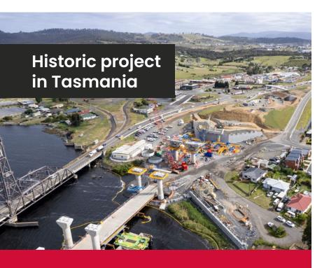
Tony Gee is delivering the design for Tasmania's largest ever transport infrastructure project - the Bridgewater Bridge replacing a 1940s lift span bridge.
